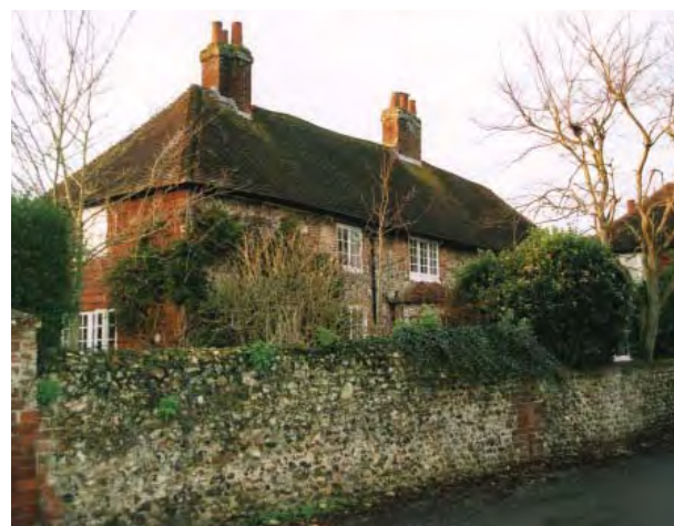
Use of flint, brick and handmade clay tiles (Apple Tree Farmhouse)
